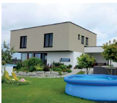
Energy Master House, Austria
